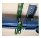
**Note:** Be sure that the trolley is placed between the two sections of the strut channel.
