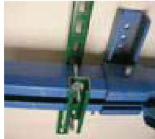
**Note:** Be sure that the trolley is placed between the two sections of the strut channel.
